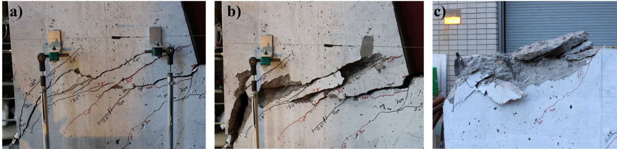
Figure 4.1-1. Damage progression for specimen 8A: (a) before sliding, (b) after concrete strength degradation, (c) after failure. (Courtesy of A. Kottari)
